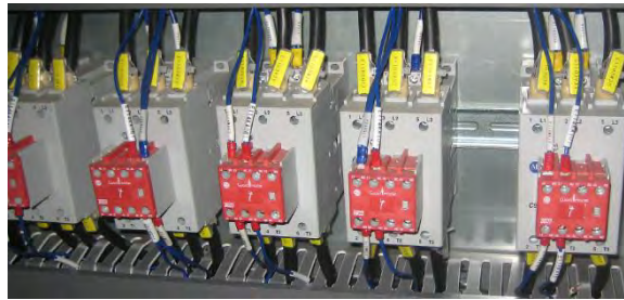
Figure 5. AB 100S-F series main contactors
